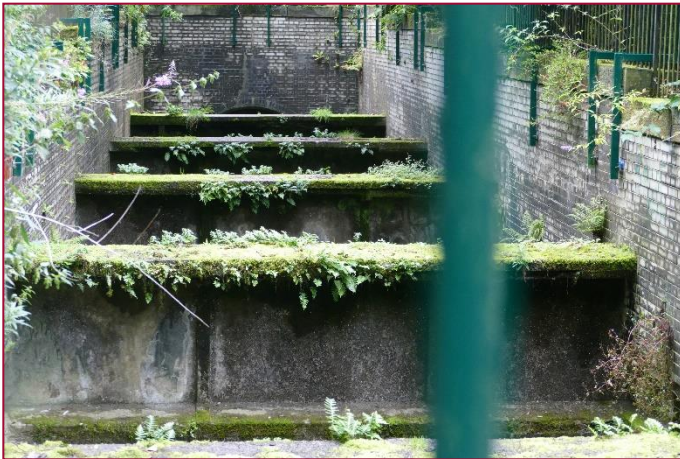
(b) The disused underground station, with suitability for roosting bats.
